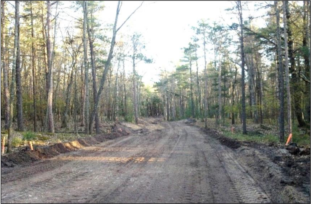
Figure 2. Common practice trail construction showing typical breadth, between Forest Haven Drive and M-109, April 2012 (Courtesy of D. Skjaerlund).
